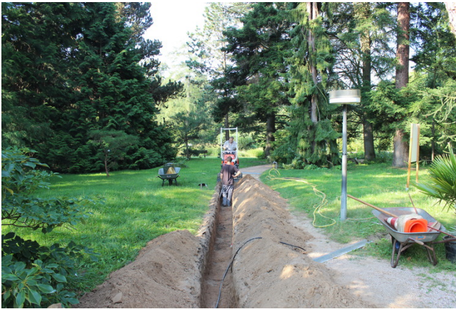
Figure 4.2: Left: The digging of the channel in which the underground power and the fiber-optic cable were placed. Right: Covering the channel.
