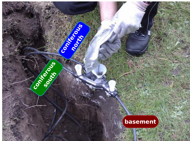
Figure 4.4: Left: Wiring the phases of the three cables. Right: Filling the branch-joint with synthetic resin.
