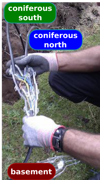
Figure 4.4: Left: Wiring the phases of the three cables. Right: Filling the branch-joint with synthetic resin.
