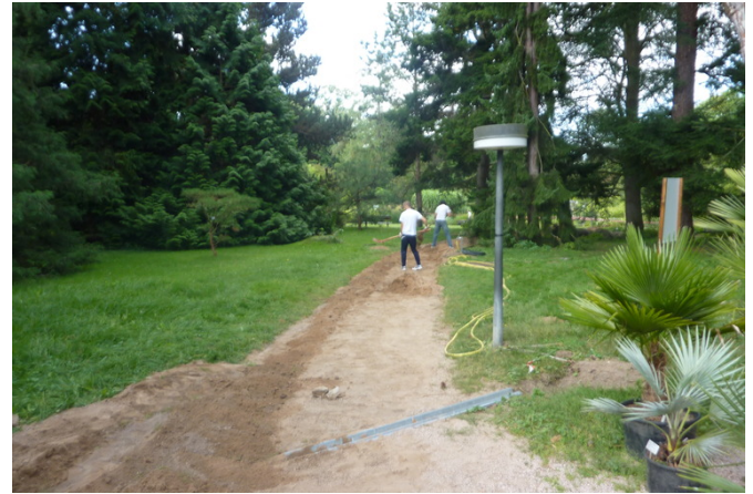
Figure 4.2: Left: The digging of the channel in which the underground power and the fiber-optic cable were placed. Right: Covering the channel.
